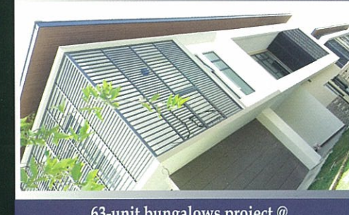
63-unit bungalows project @ East Ledang, Nusajaya, J. Bahru
