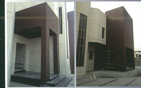
external wall cladding @ Qatar
