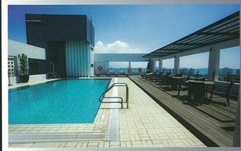
Roof Top Pool Deck (Condominium) @ Penang
